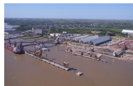
The construction of the new terminal employed more than 600 construction workers
