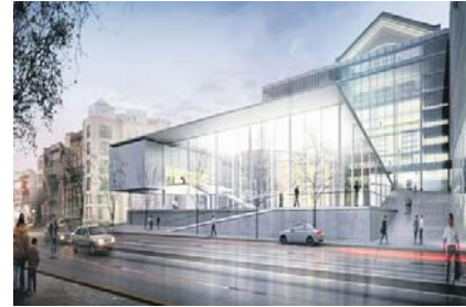
The intelligent building of BROU will demand an investment of USD 50million
